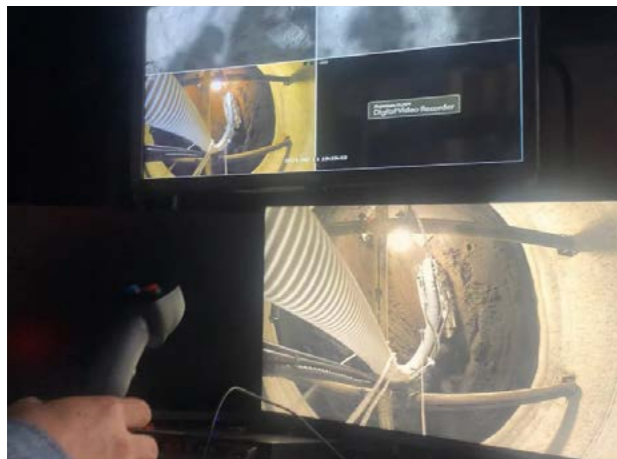
Robots employed in high-risk nitrogen work
